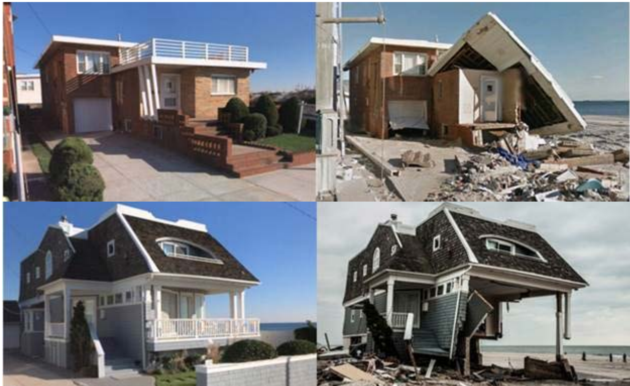
Figure 2-4: Before and After Photos of Rockaway Beach Structures Damaged by Hurricane Sandy
