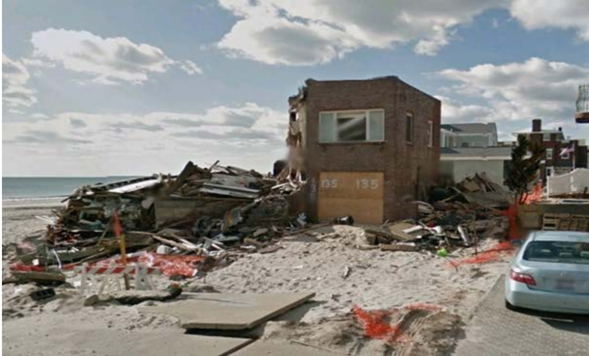
Figure 2-3: Rockaway Beach Structure Damaged by Hurricane Sandy
